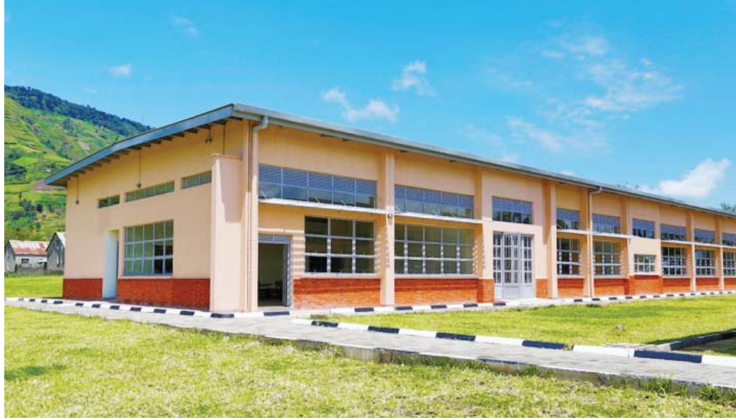
A newly built Welding and metal fabrication workshop at UTC Kichwamba, Kabarole district.
