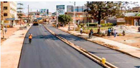
Construction Of Ntinda Road
